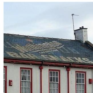
**Figure 15.14.120-9:** Roof Sign, Integral
