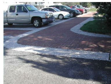
Figure 15.14.060-9: Change in paving materials to distinguish pedestrian walkway
