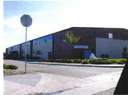
Figure 15.08-25: Image of typical development in the I-1 zone district.
