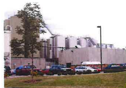
Figure 15.08-26: Image of typical development in the I-2 zone district.
