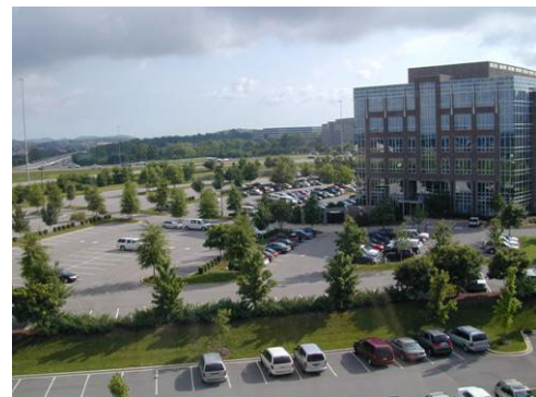
Figure 15.08-31: This example shows a parking lot with landscaped areas separating parking groups.
