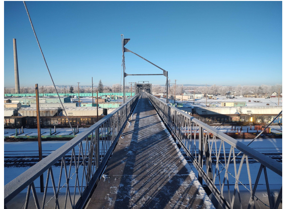
Figure 12: Garfield Footbridge over UPRR Rail Yard
